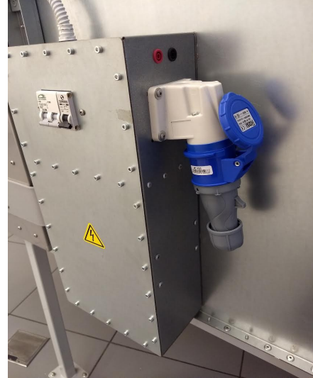
Line filters box
